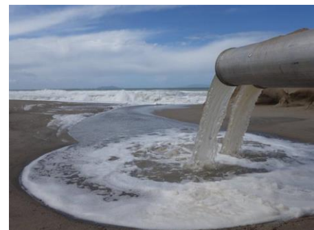
Figure 4 – Storm water drains into the Pacific Ocean at Oxnard Shores neighborhood
