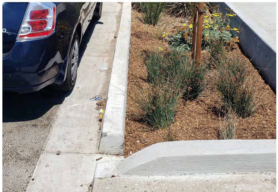
Curb extensions with low-level planting or bioswales increase greening and create a buffer between cars and people walking. Source: City of Oxnard
