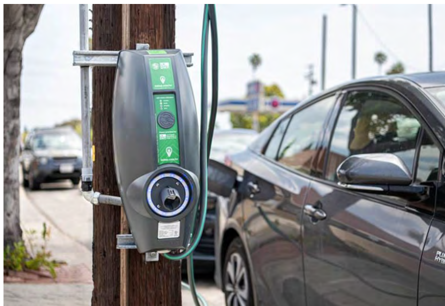
EV Charger on streetlight pole. Source: Los Angeles Cleantech Incubator (LACI)
