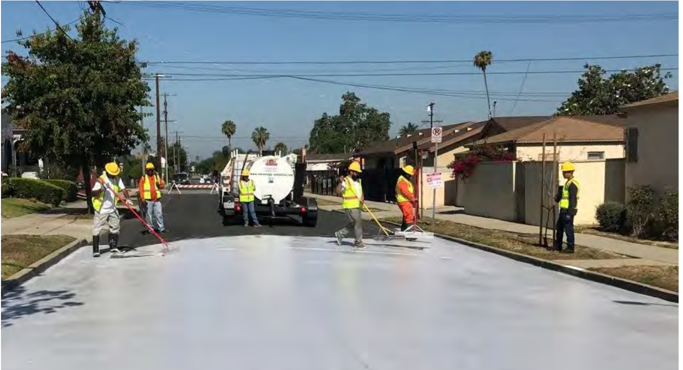
A light gray cool pavement coating applied in Los Angeles was found to have a 10-degree reduction in heat. Source: New York Times
