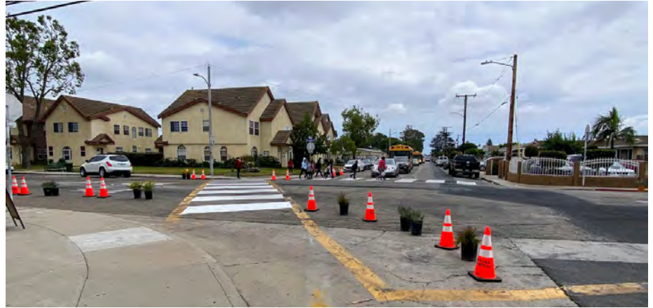
Demonstration Project 1 at Juanita Avenue & Colonia Road illustrated how a bulbout (temporarily made with cones and plants) could slow down vehicles, improve pedestrian visibility, and shorten pedestrian crossing distances
